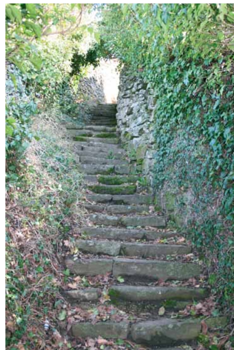
Figure 10: Long stone stairs between the dry stone walls of the terraces. Slika 10: Dolge kamnite stopnice med suhozidi teras.
