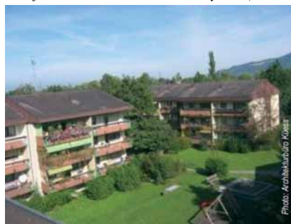
Slika 7: Zunanost stanovanjskih objektov Dornbirnu pred prenovo. Vir: Task: 37, Architecturbüro Kuess, www.iea-shc.org/task37 Figure 7: Exteriors of housing structures in Dornbirn before renovation.
