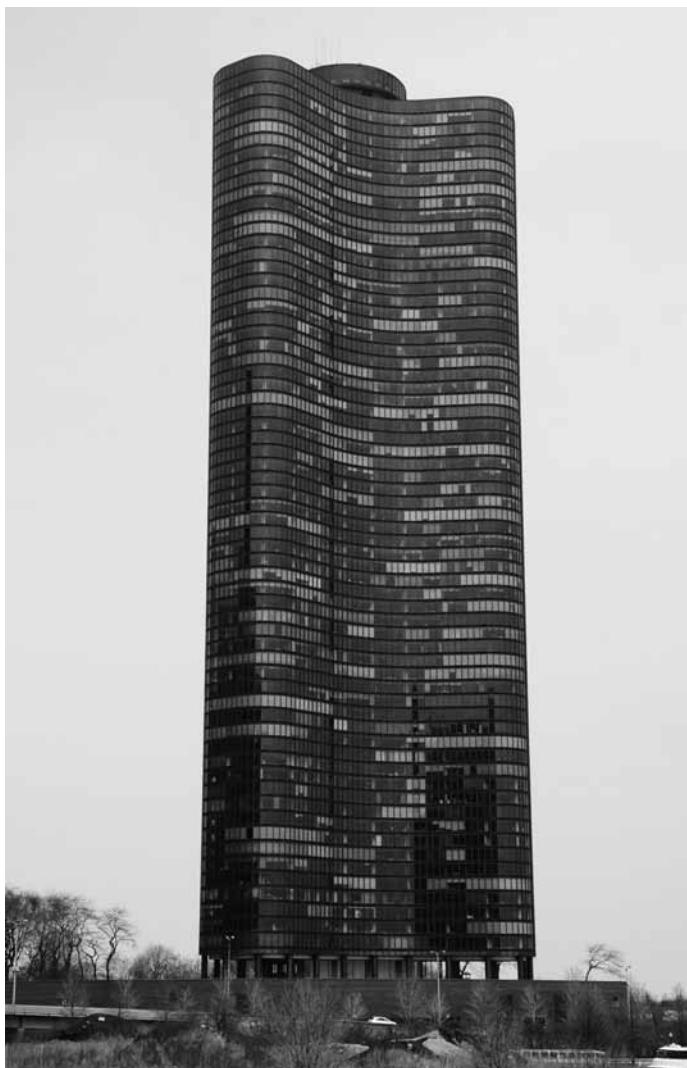
Slika 10: Schipporeit & Heinrich: Lake Point Tower, 1968. Figure 10: Schipporeit & Heinrich: Lake Point Tower, 1968.
